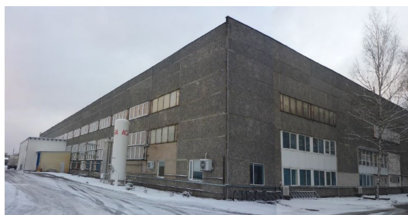
Production building before project implementation
